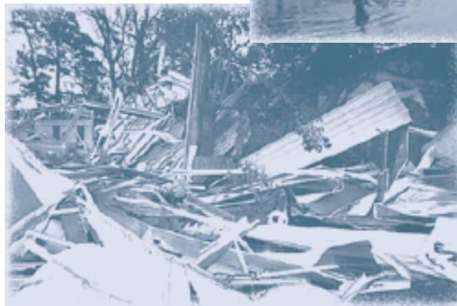
Hurricane Katrina caused massive destruction and catastrophic flooding in the Gulf Coast areas.
